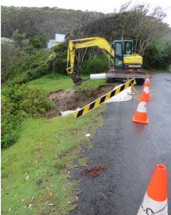
Figure 9. Aquares for land was utilised to investigate the root cause of a road slip in Seal Rocks, NSW.
